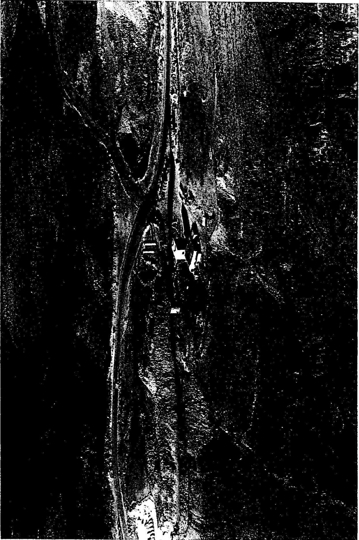
GYPSUM MINE SITE OFFICES
