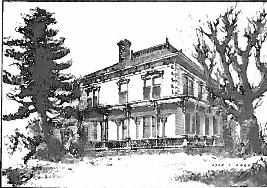
LAKE MANSION, S. VIRGINIA ST. AT CALIFORNIA, RENO
