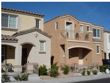
A variety of architectural features (including colors and styles) contributes to the overall aesthetic quality of a neighborhood.
