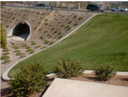
A well-designed storm drainage area will protect other areas of the city.
