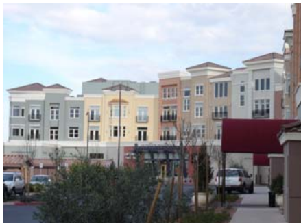
Nearby housing helps generate enough activity to support transit.
