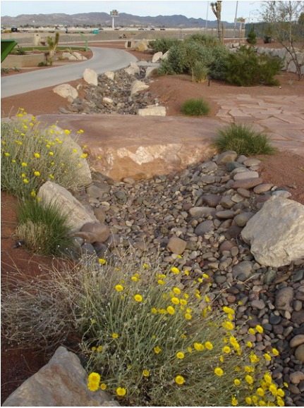
Integration of trails, proper drainage, and desert landscaping conserves resources and offers aesthetic value.
