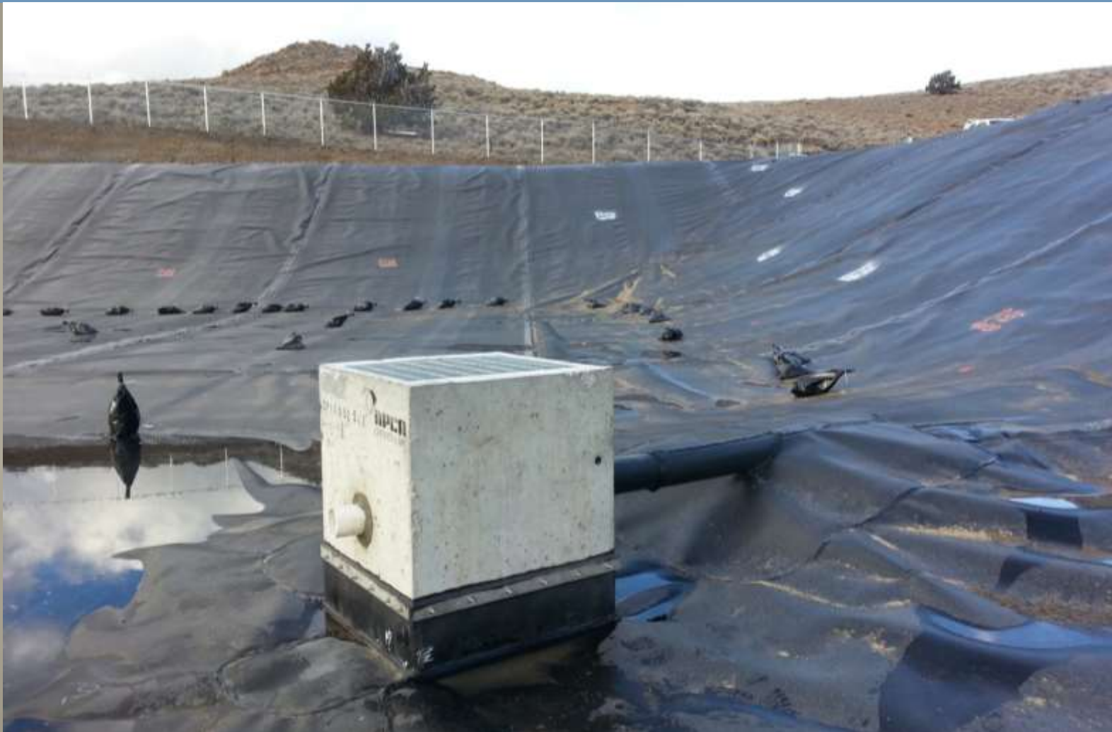
5-Mile Reservoir – Outlet Structure
