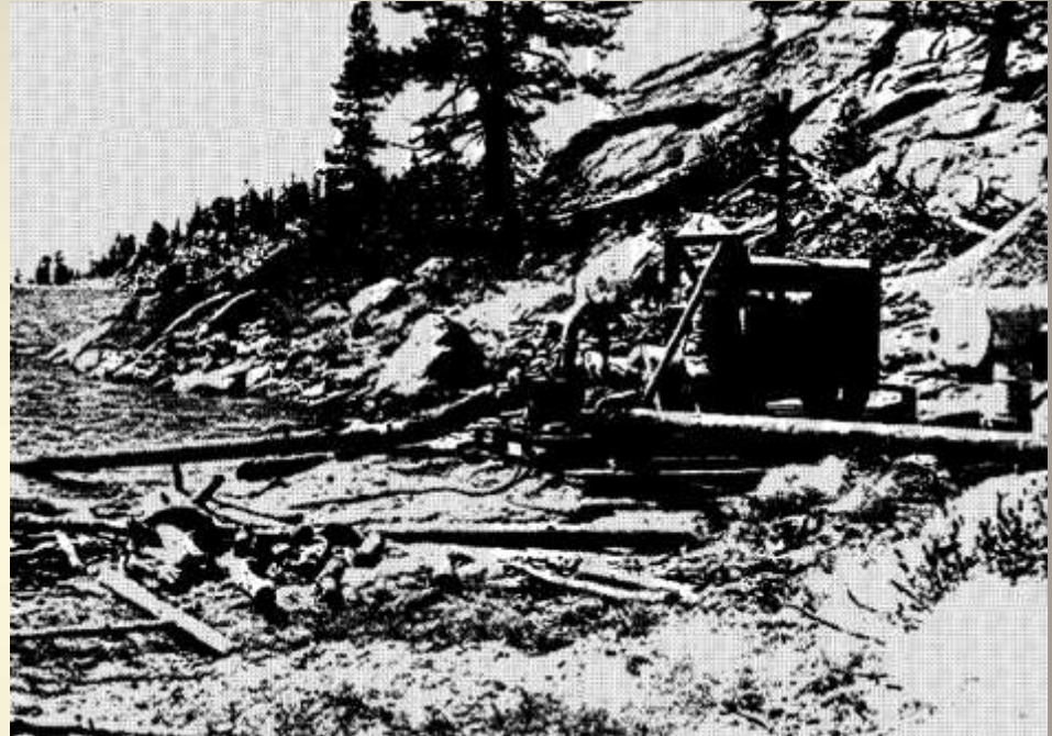
Marlette Lake – Pump Station (1968)
