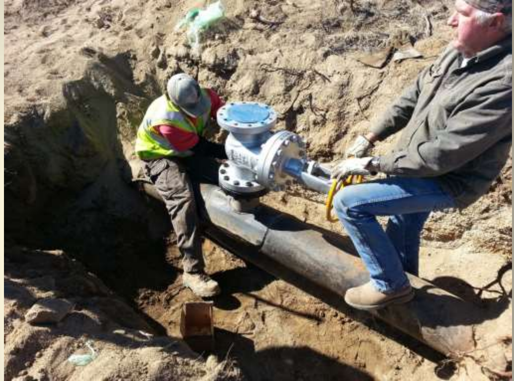
High Pressure Valve being Installed
