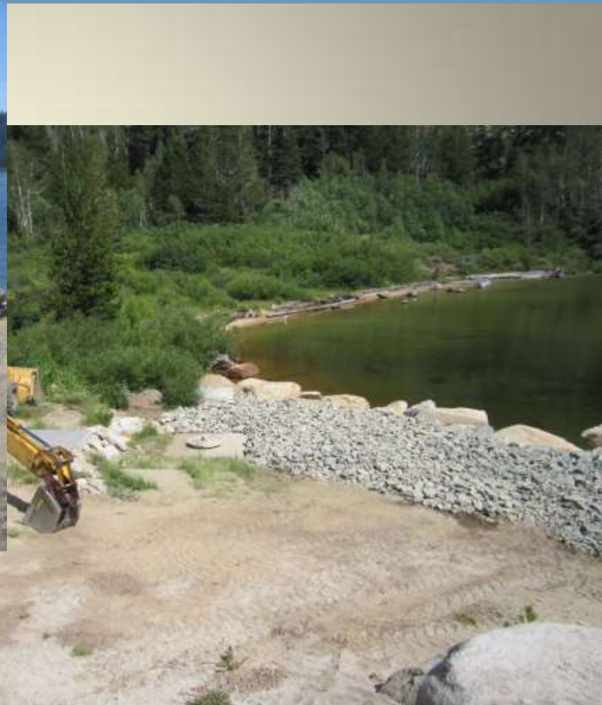
Marlette Lake Pump Site After Site Rebuild
