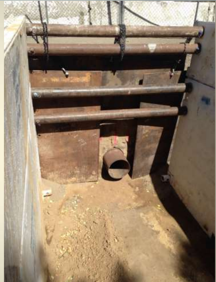
New Pipe Sleeve Installation Under I-580
