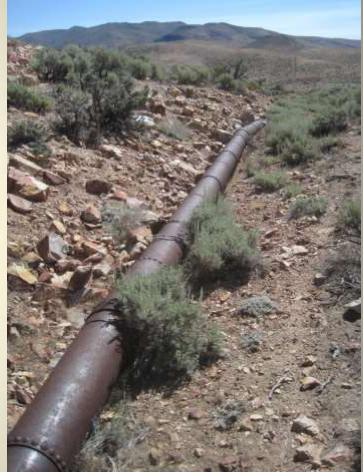
Pipeline-1 (Riveted Pipe)
