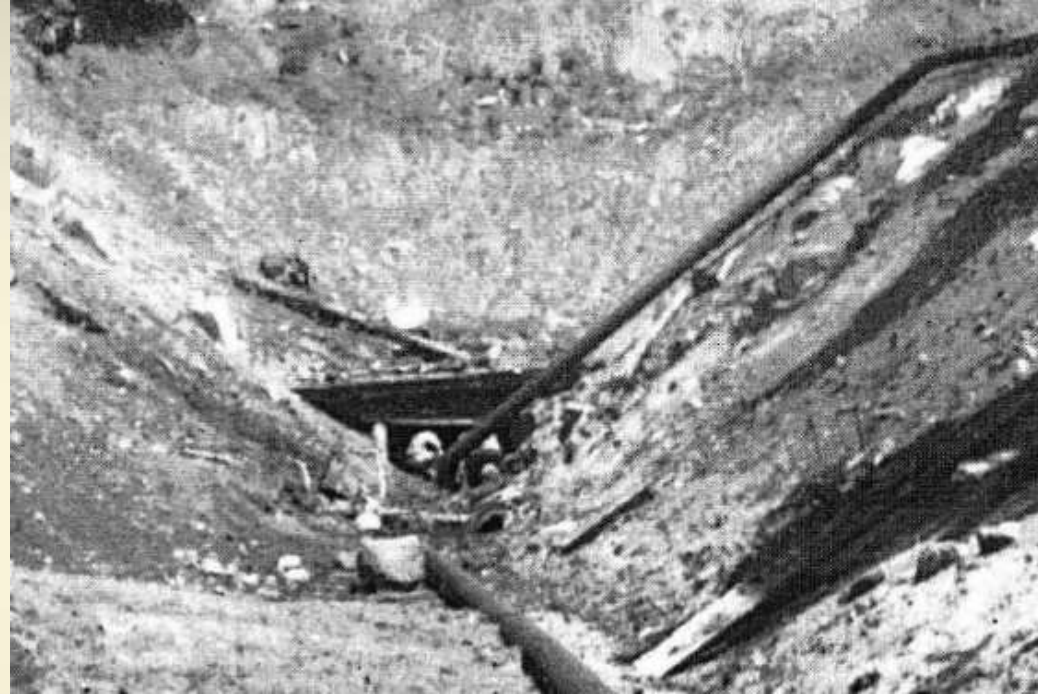
West Incline Tunnel Portal, 1968
