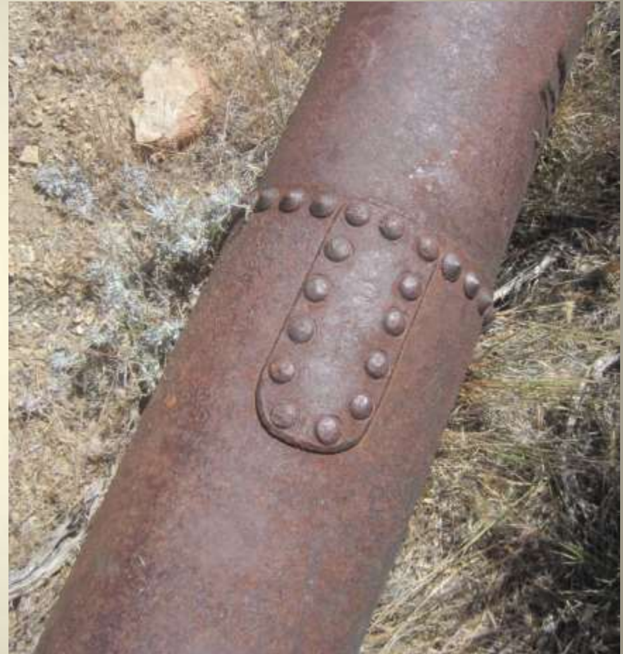
Pipeline-1 (riveted)
