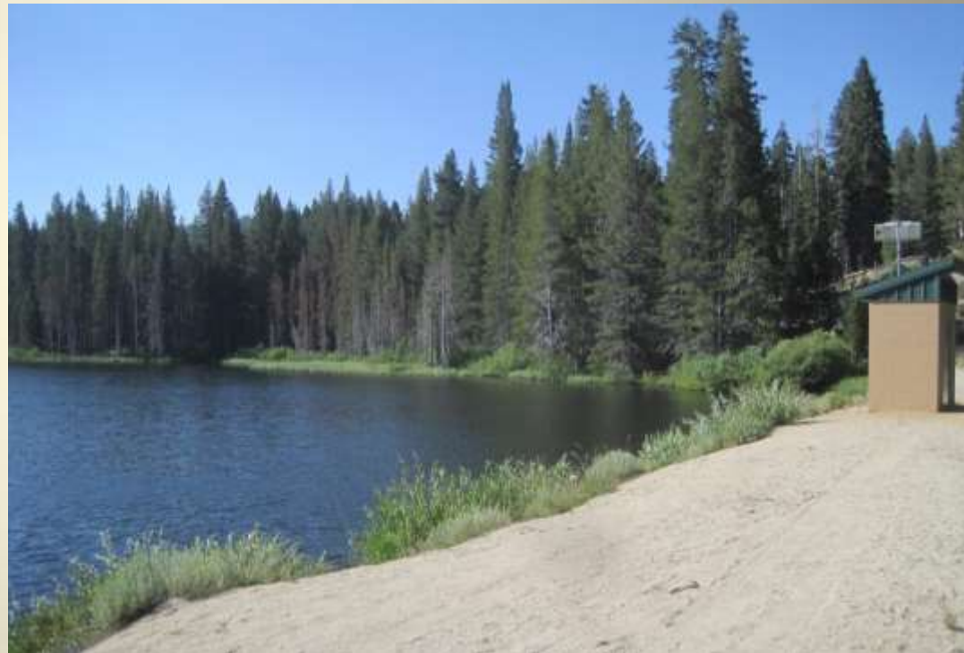
Hobart Reservoir Dam – Outlet Control Building
