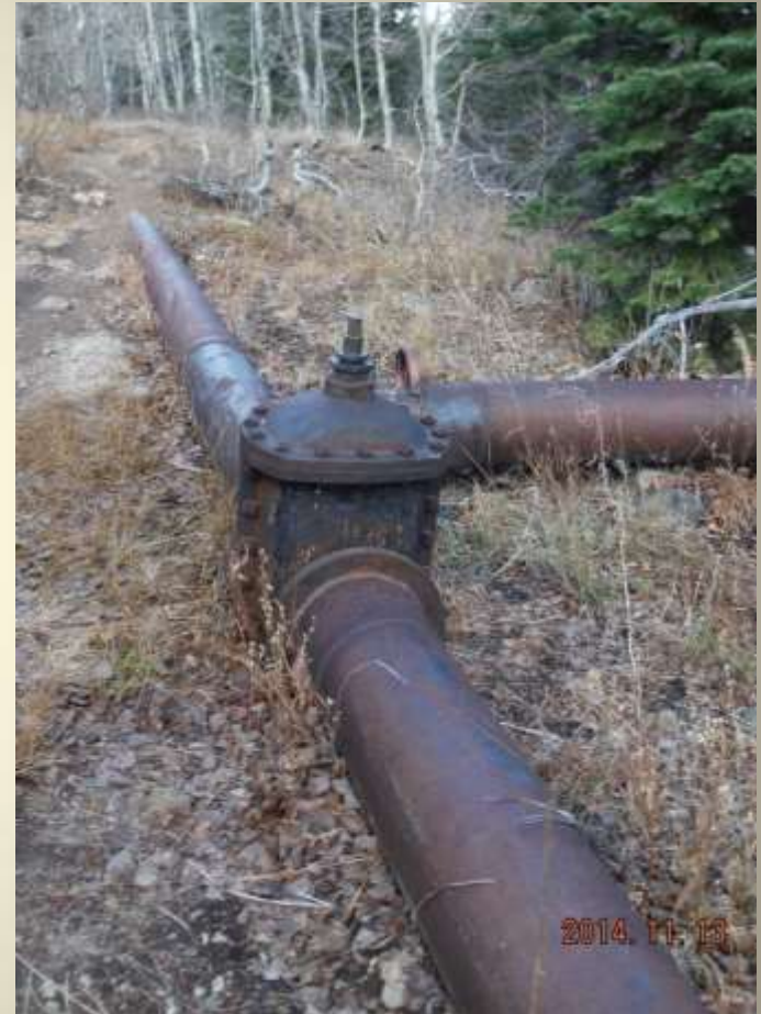
East Slope Pipeline (Near Diversion)
