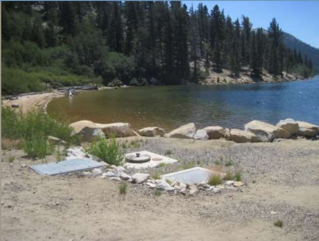
Marlette Lake Pump Site Before Erosion
