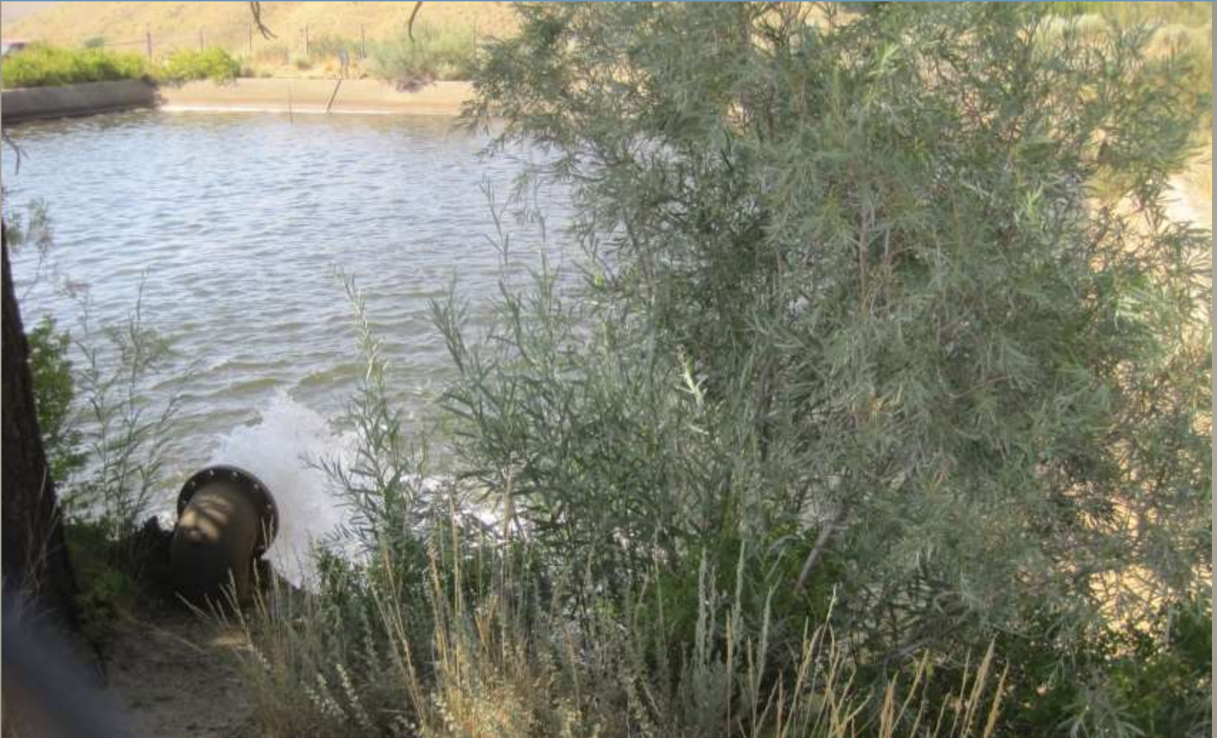
1MG Concrete Reservoir – from Air Box-3
