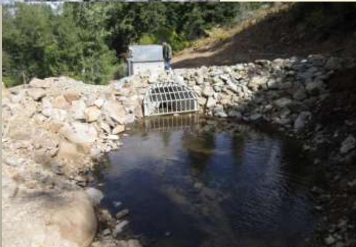
Catchment #6 Inlet Showing Reshaped Inlet Bowl to Improve Runoff Collection
