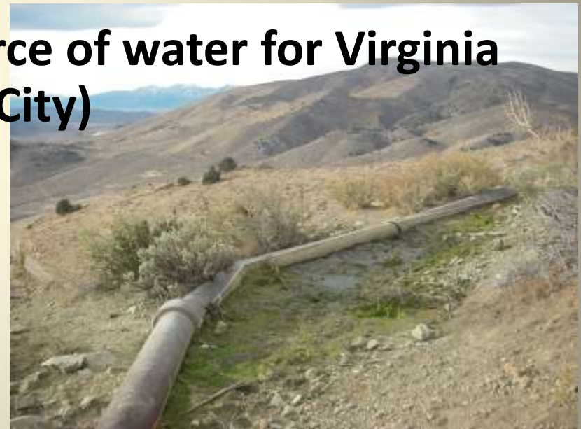
10" dia. lead joint pipe
