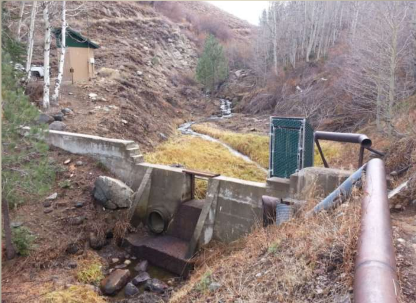
Diversion Dam – Prior to Work Project in 2017
