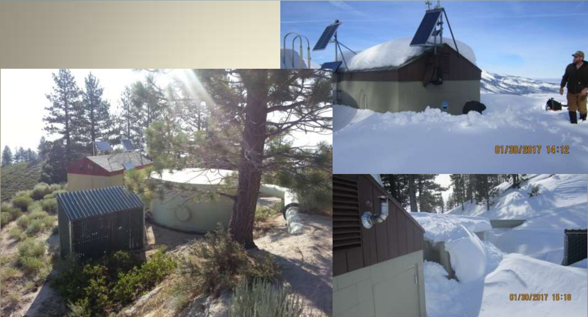
Lakeview Tank Site and Control Building
